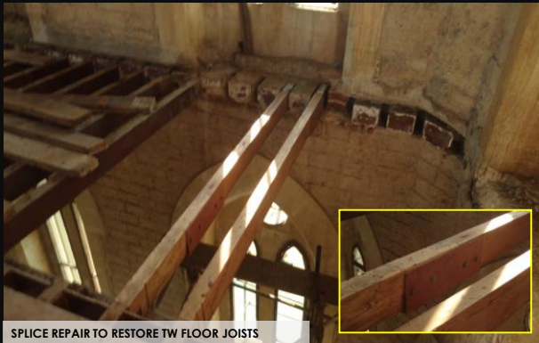
SPLICE REPAIR TO RESTORE TW FLOOR JOISTS
