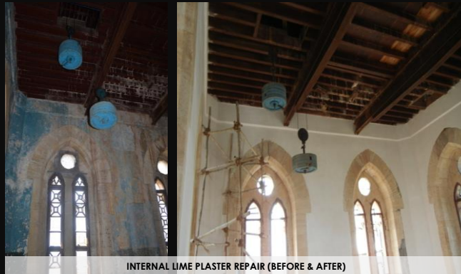
INTERNAL LIME PLASTER REPAIR (BEFORE & AFTER)
