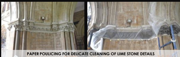
PAPER POULICING FOR DELICATE CLEANING OF LIME STONE DETAILS
