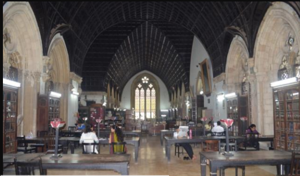
LIBRARY BURMATEAK CEILING RESTORATION
