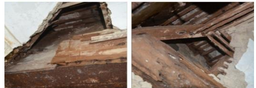
FIRST FLOOR FRAMEWORK IN STEEL GIRDERS WITH BURMA TEAK LATH PLASTER SURFACE STEEL FOUND RUSTED, IN DIRECT CONTACT WITH LIME
