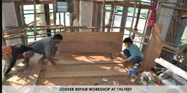
LOUVER REPAIR WORKSHOP AT 196 FEET
