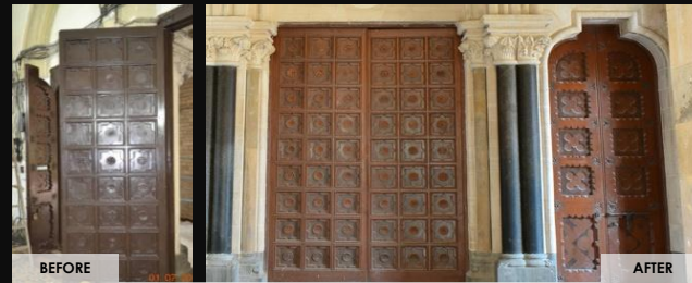
DOORS & WINDOWS RESTORATION REMOVAL OF PAINT & POLISHING
