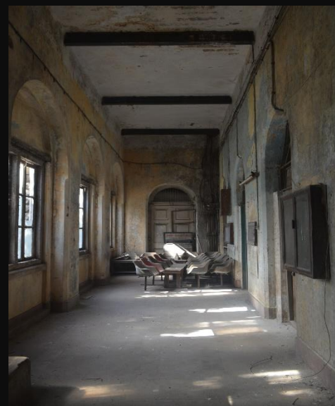
First Floor Balcony
