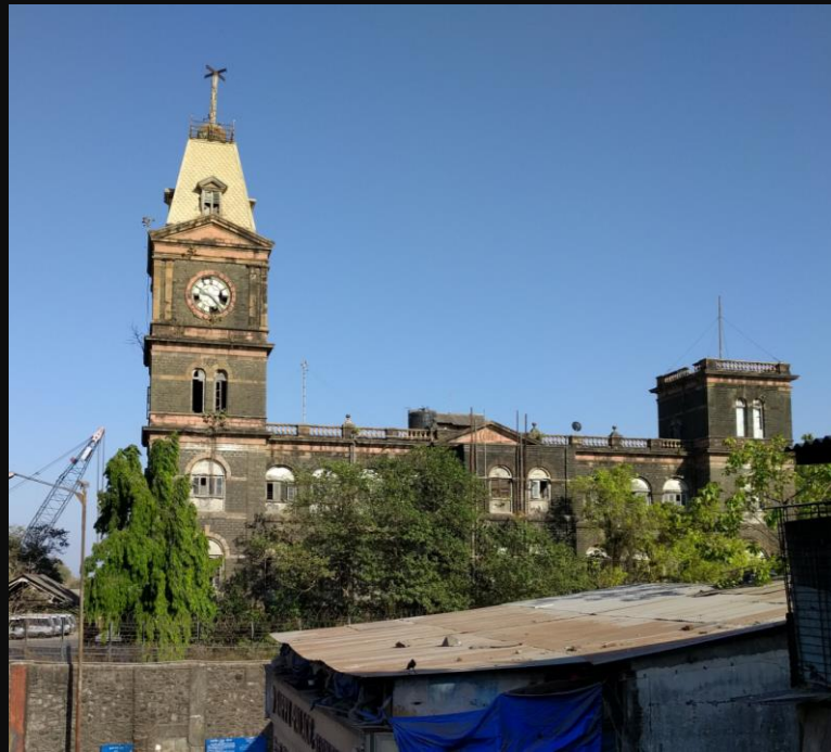
Traffic Office (Time ball Building) at Prince's & Victoria Dock
