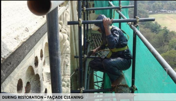
DURING RESTORATION – FAÇADE CLEANING
