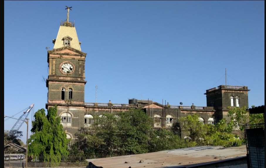
Traffic Office (Time ball Building) from P D'Mello Road
