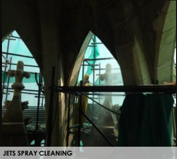
JETS SPRAY CLEANING
